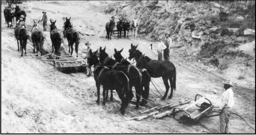
FIGURE 16. Road work around 1914, probably between Lubbock and Farwell. Vic Barber (1).
