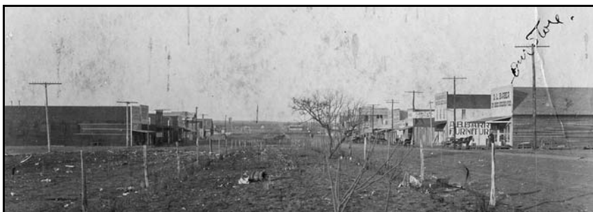
FIGURE 8. Lee and Johnny's store on the north side of Snyder Avenue, about 1908. Cleveland Avenue separates them from the A B Barrow Furniture Store.
